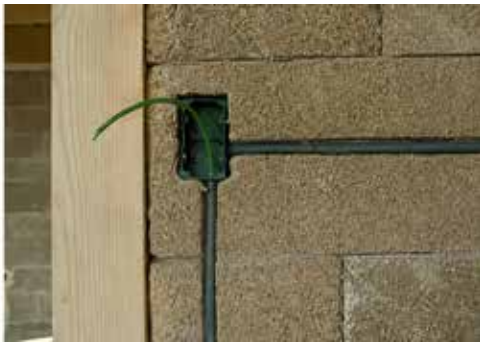
Chase in Biomattone® for electrical system
