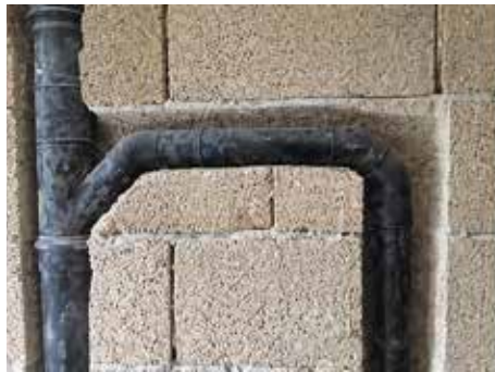
Chase in Biomattone® for plumbing system
