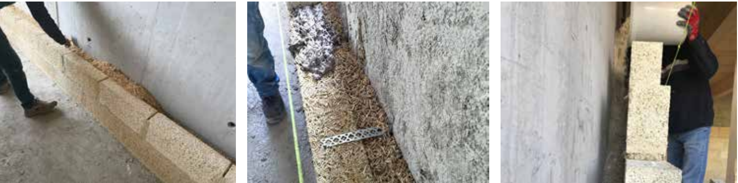
Inner lining in Biomattone® with cavity filled with Biobeton
