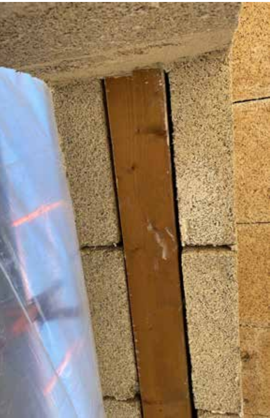
Installation of a kiln-dried timber lintel on a Biomattone® wall with thermal bridge resolved
