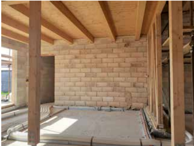
Internal partition wall in Biomattone®
