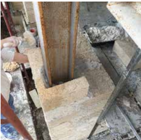
Shaped Biomattone® used to resolve a thermal bridge at the structural frame
