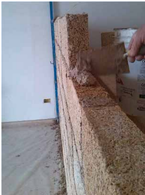
Installation spreading a layer of Malta Pronta
