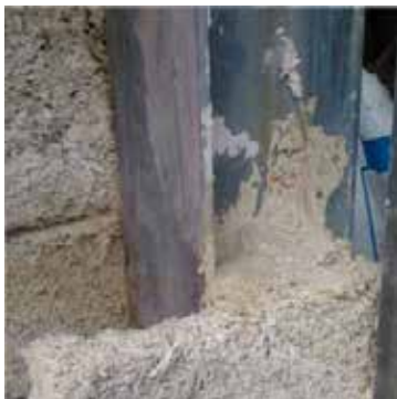
Biomattone® shaped block used to solve the thermal bridge from the structural frame
