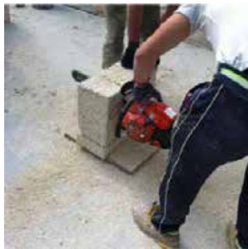
Biomattone® cutting with electric chain saw
