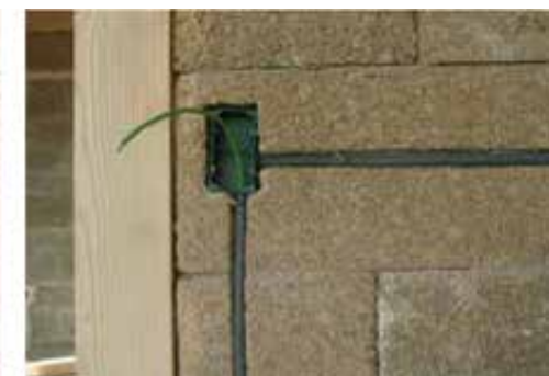
Grooves on Biomattone® for electrical system
