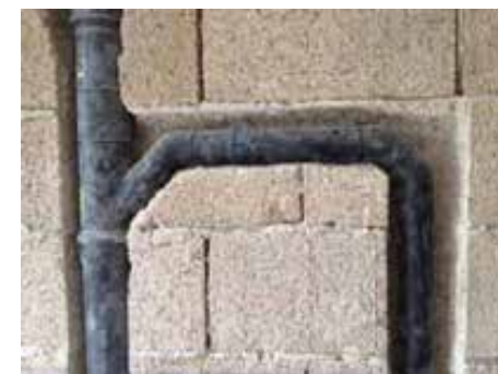
Grooves on Biomattone® for sanitary system
