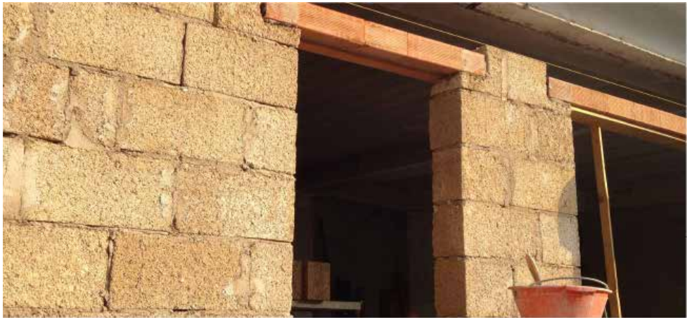
Installation of a clay lintel on a wall made of Biomattone®
