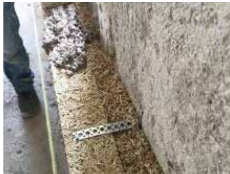
Counterwall of Biomattone® with a cavity filled with Bio Beton®200 Pronto
