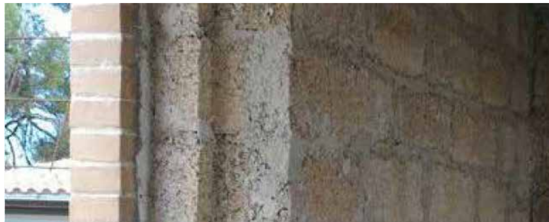
Shaping of the Biomattone® for housing the basic frame made on site
