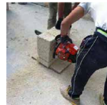
Biomattone® cutting with electric chain saw
