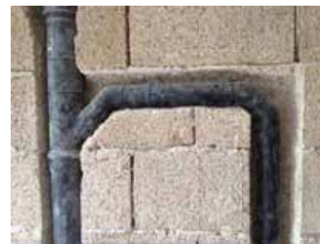
Grooves on Biomattone® for sanitary system
