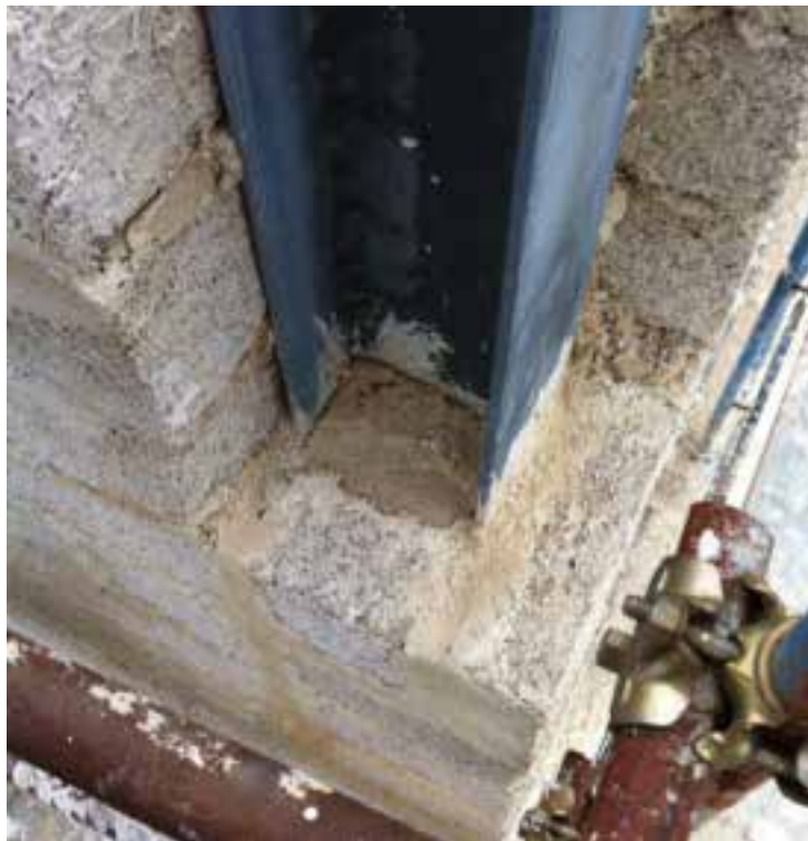
Steel frame: Thermal bridge correction with Biomattone® shaped at the corner column
