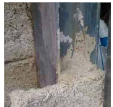
Biomattone® shaped block used to solve the thermal bridge from the structural frame
