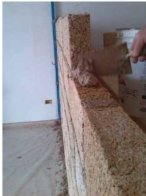
Installation spreading a layer of Malta Pronta
