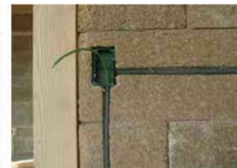
Grooves on Biomattone® for electrical system
