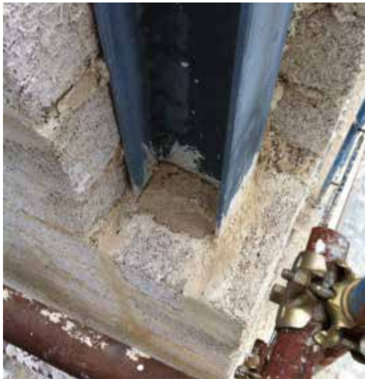
Steel frame: Thermal bridge correction with Blocco Ambiente® shaped at the corner column
