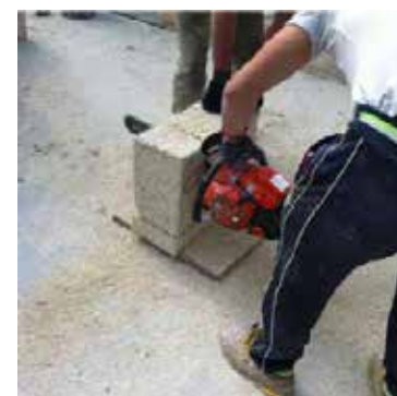
Blocco Ambiente® cutting with electric chain saw
