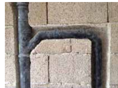
Grooves on Blocco Ambiente® for sanitary system
