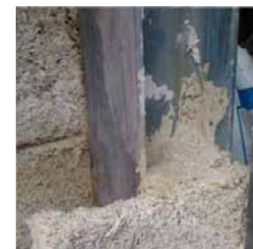
Blocco Ambiente ® shaped block used to solve the thermal bridge from the structural frame
