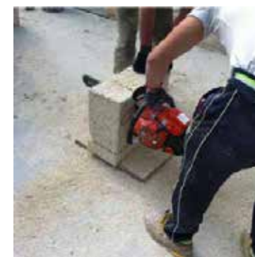
Blocco Ambiente ® cutting with electric chain saw
