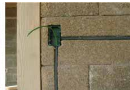
Grooves on Blocco Ambiente® for electrical system
