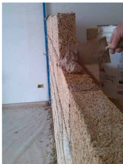
Installation spreading a layer of bedding mortar
