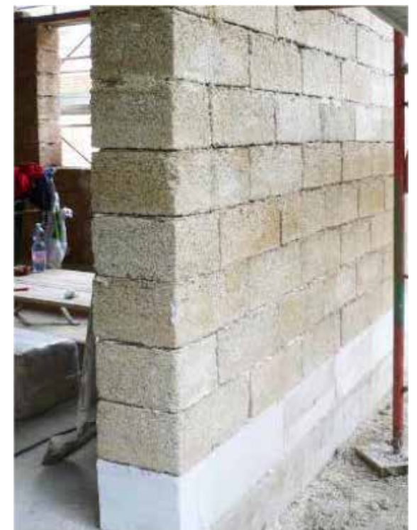
Insulation of the first course with cellular glass
