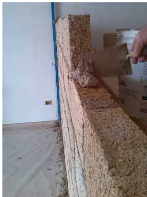
Installation spreading a layer of bedding mortar
