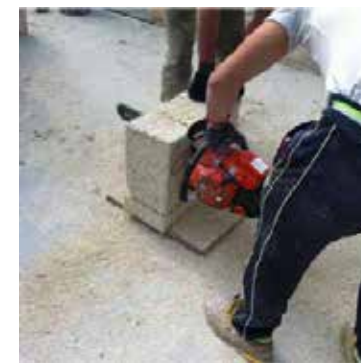
Blocco Ambiente ® cutting with electric chain saw
