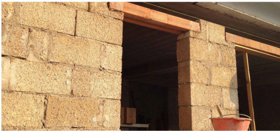
Installation of a clay lintel on a wall made of Blocco Ambiente®
