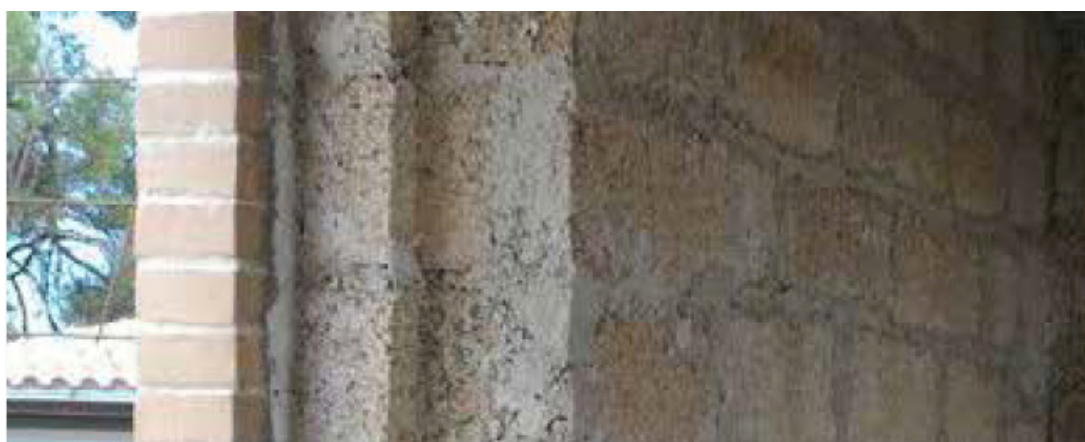
Shaping of the Blocco Ambiente® for housing the basic frame made on site
