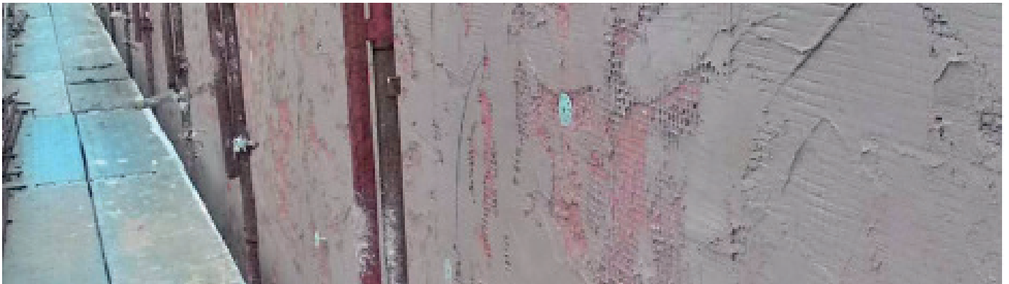
Application of an overcoat mesh with a first coat of Stabilitura Naturale Traspirante Plus
