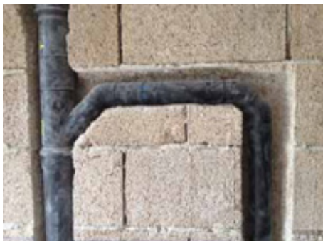
Grooves on Blocco Ambiente ® for sanitary system
