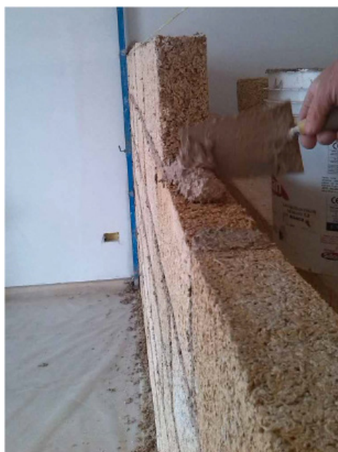
Installation spreading a layer of bedding mortar
