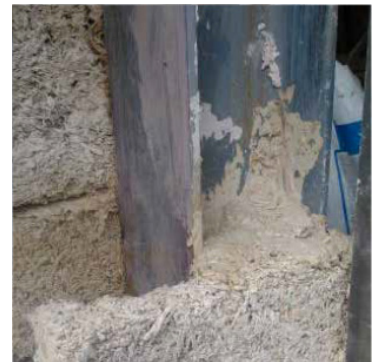
Blocco Ambiente ® shaped block used to solve the thermal bridge from the structural frame
