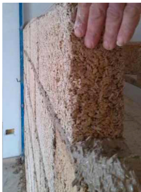
Installation spreading a layer of bedding mortar
