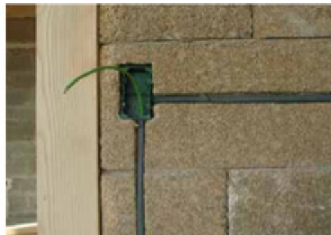
Grooves on Blocco Ambiente ® for electrical system
