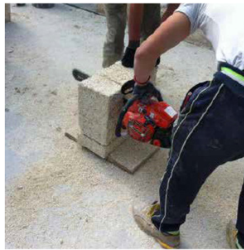
Blocco Ambiente ® cutting with electric chain saw
