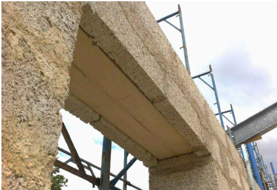
Installation of a dried wood lintel on a wall in Blocco Ambiente® including the correction for thermal bridges
